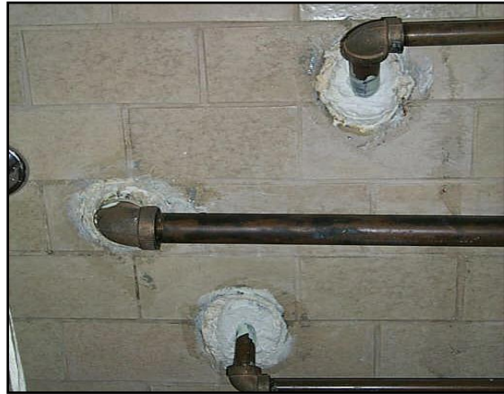
Figure 2: Filled poke-throughs
