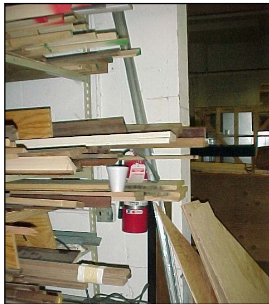
Figure 5: Inaccessible fire extinguisher
