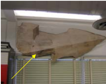
Figure 1: Dark Mold Growing on Water Damaged Wall behind Wall Paper
