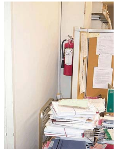
Figure 1 Fire extinguisher obstructed from view and not easily accessible.
