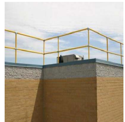
Fig. 1: Guardrails along roof edge
