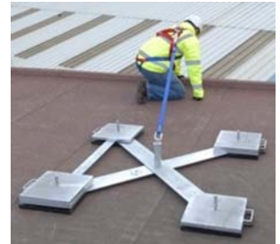
Fig. 5: Fall Restraint System
