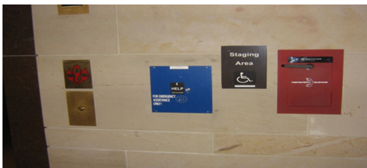
Image 4: Staging area for emergency evacuation with two way communication unit.
