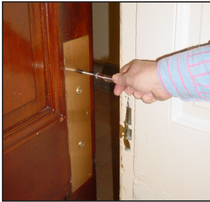
Figure 4: Testing restroom door weight
