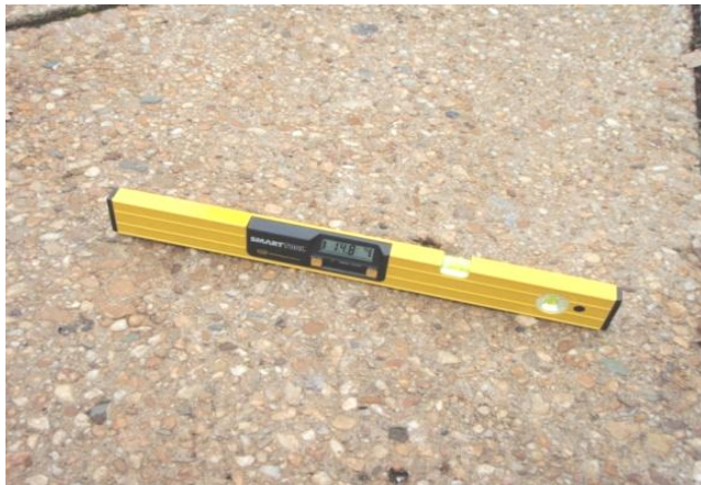
Level Measuring Curb Cut Slope at 14.8%
