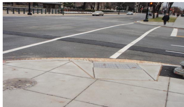
Curb Cut Outside of Marked Cross Walk
