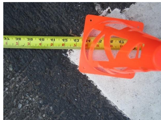
Close-up of Tape Measure in Previous Photo (Curb Ramp 16)
