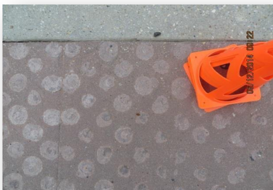
Figure 4. Deteriorated detectable warning domes on a curb ramp located on the southwest side of Capitol Building.
