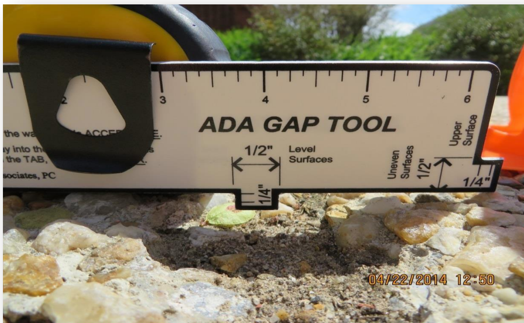
Figure 6. A Capitol grounds expansion joint gap measurement.
