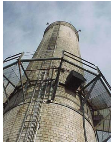
Lightning protection systems at the plant were upgraded in response to an OOC citation.
