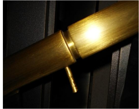
Picture 1: Brass Connector Pin Protruding From Handrail
