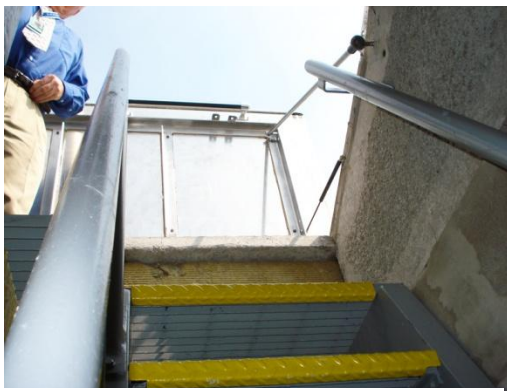
Picture 3: Example Of An Excellent Solution To A Fall Hazard
